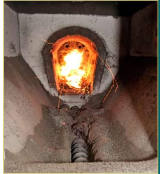
The pellet boiler has two adjoining chambers. First is a stoker, with air holes through which fans force air while an auger pushes in fuel pellets. Ignition in the stoker creates a very hot fire that is blown into the second chamber, the firebox. In high-fire mode, the boiler runs at 900-1,200 degrees Fahrenheit, with a surrounding water jacket regulating the temperature.
