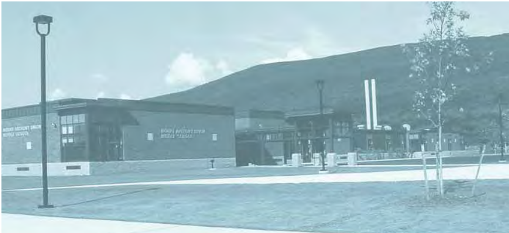
At Mount Anthony Union Middle School, heating system operators now spend only 20 minutes a day with the wood heating system.
